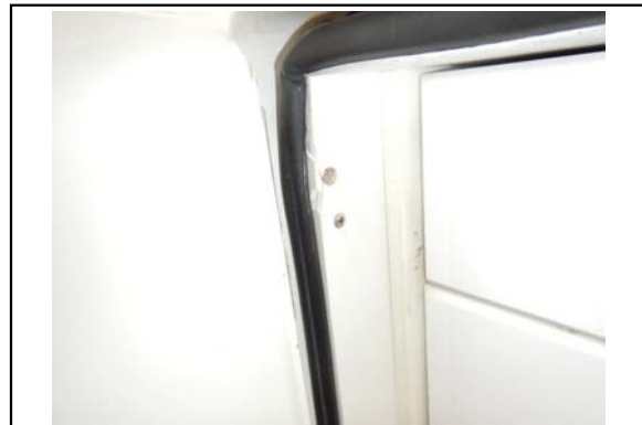
CRACKED FRAMEWORK
