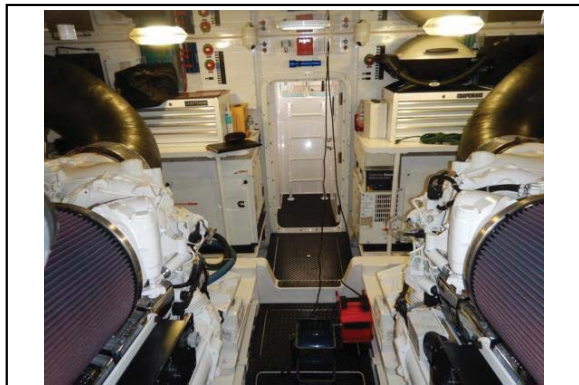
ENGINE ROOM CTR AFT
